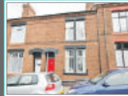
Prescot Road, St Helens £75,000 • Three Bedroom Mid Terrace House • Deceptively Spacious • Convenient For Town Centre Access • UPVC Double Glazing
